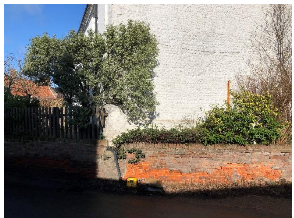
Figure 3.9: Vibration Monitor at Whitehouse Farm
