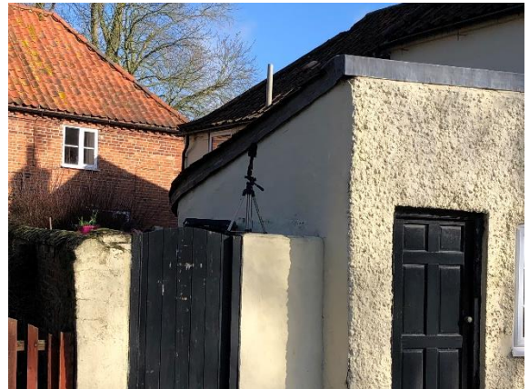
Figure 3.3: Sound Level Meter at 20 High Street
